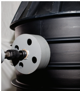
Drill a hole for a LKS inlet gasket
