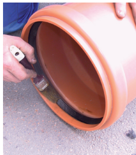
... and the PVC pipe and gasket
