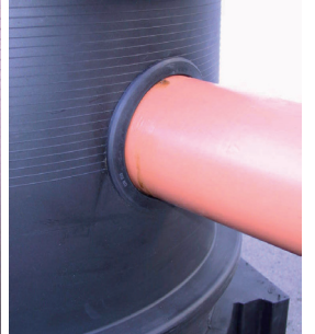
Connect the PVC pipe
