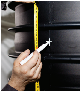
Determine the medium height of the additional connection
