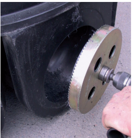
Drill the inlet with suitable hole saw cup, adapter, adapter and handheld drilling machine
