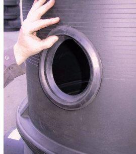
Insert the KS inlet gasket
