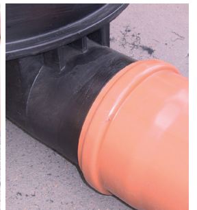
Attach the PVC pipe
