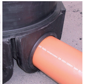
Attach the pipe to the chamber
