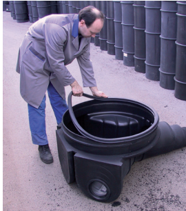
Attach and lubricate the gasket
