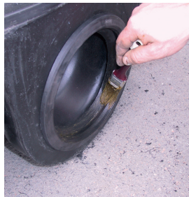
Lubricate the inlet gasket and PVC pipe
