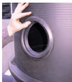
Install the inlet gasket
