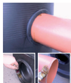
Connect the PVC duct pipe
