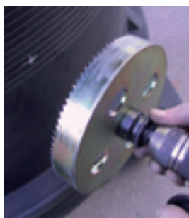
Drill a hole for inlet gasket
