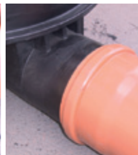
Attach the PVC pipe
