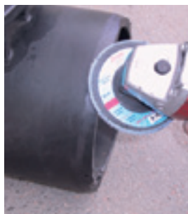
Cut off the rim for 15 mm/30°
