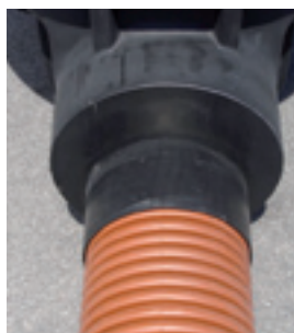
Properly lubricate the interior of the connection and the gasket, push the pipe into the chamber
