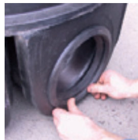
Install the inlet gasket
