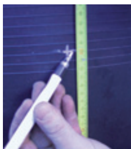
Mark the centre point of additional inlet
