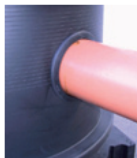
Connect the PVC pipe
