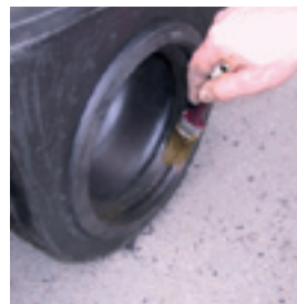
Lubricate the inlet gasket and PVC pipe
