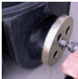
Drill the inlet with suitable saw, adapter and handheld drilling machine
