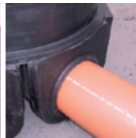
Attach the pipe to the chamber
