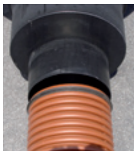
Place gasket on pipe (according to instructions by the pipe manufacturer)
