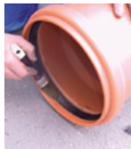
... and the PVC pipe and gasket
