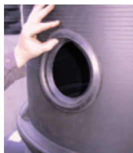
Attach the gasket
